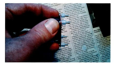
Now here's the eye-hand coordination part: Push the screws through the holes in the bottom of the project box (without losing the plastic tubes!) NOTE: The screw terminals face the bigger hole. When they're through the holes in the bottom, put the nuts on the ends of the screws and tighten. If the screws don't stick out far enough, you may need to trim the plastic tube sections a bit.
